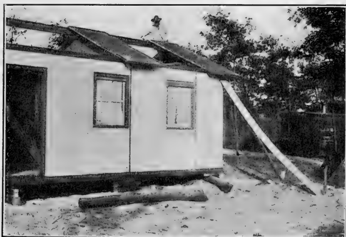
Erecting the portable house
